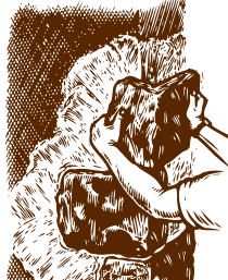
FIG. 5 Install Corners First
