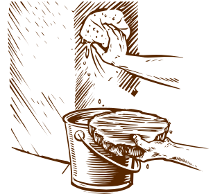
FIG. 3 Wet the Scratch Coat and Veneer
